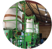
Resin Fill Operations
